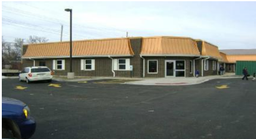
Mid Lakes Clinic expansion, Lake County Health Department, 224 W. Clarendon Drive
